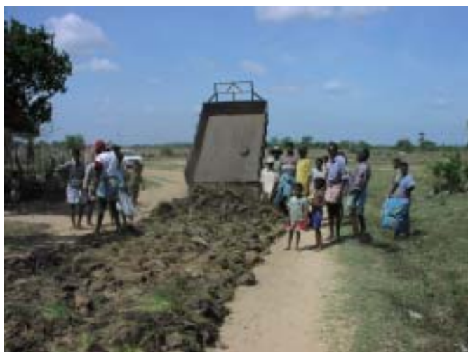
Clay is spread on the new road: Food-for-work for road construction between Ilankaithurai and Eachchilampattai
