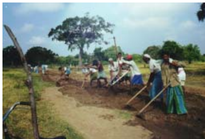
Access road to paddy fields: Food-for-work project in Pulmoddai
