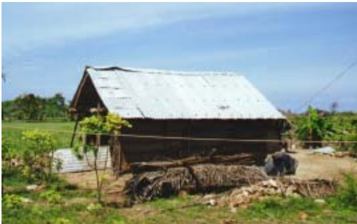
A new and longer lasting roof
