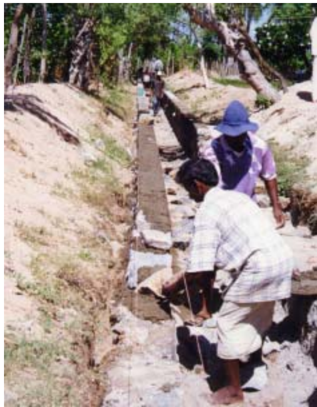
Constructing the storm water drainage system in Gopalapuram
