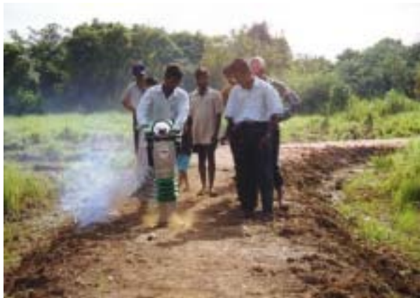
Compacting the bund
