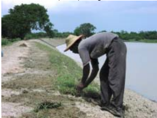
Turfing: Protection against erosion
