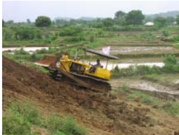
Earth works: sloping the bund
