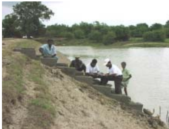
Bathing steps under construction
